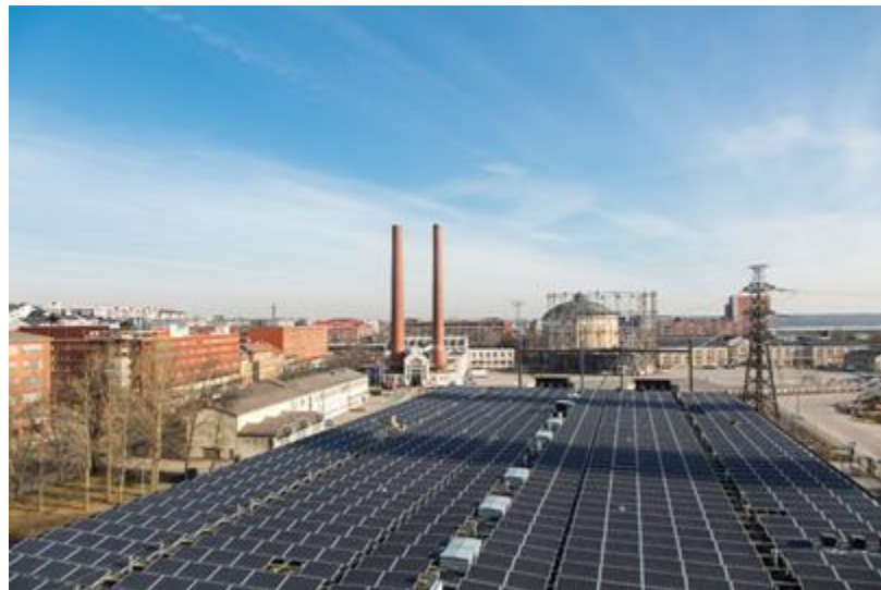
Solar power plant in Suvilahti
